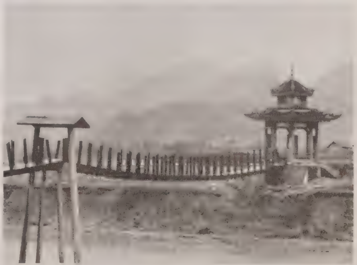
Footbridge over a channel in the Tu Chiang-yen irrigation system on the Ch'eng-tu Plain, Szechwan Province.
